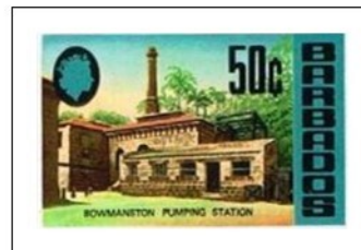
Bowmanston Pumping Station
